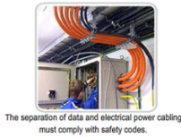
The separation of data and electrical power cabling must comply with safety codes.
